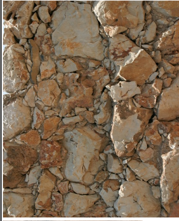
Picture 4: Apparent fire damage to Hazor
